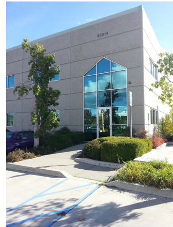
Postage One building located in Valencia, CA
